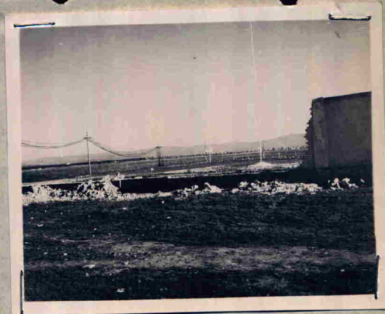
Part of the wall that was torn down to use the limestone blocks for the construction of huts to house the officers of the 301st Bomb Group Hdqs Sq. Each hut will house four men complete with stove, cement floor and white washed walls.
