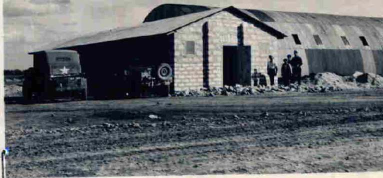
The new briefing room for the 301st Bomb Group as it nears completion. The attachment in the rear of the briefing room is for the S-2 and S-3 offices. A large stage is also being constructed to insure room for the future USO shows that will be in this area.
