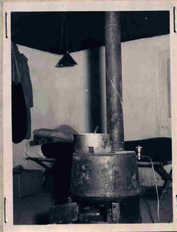
Partial view of one of the completed huts that will house four men for hdqs Sq. 301st Bomb Gp.
